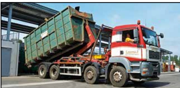
When full, the containers can be removed from ground level by hooklift trucks without having to close the site to public on the deck level.
