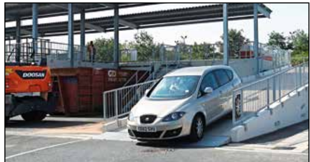
Job done... residents enter and leave the deck by ramp sections that are part of the Modulo-Beton “kit”.
